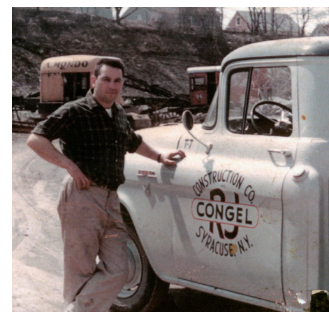
Robert J. Congel starts his career as a construction contractor in Syracuse New York
